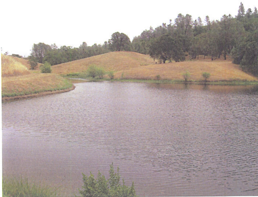
Reservoir named in Permit 18997 Standing on dam looking upstream
