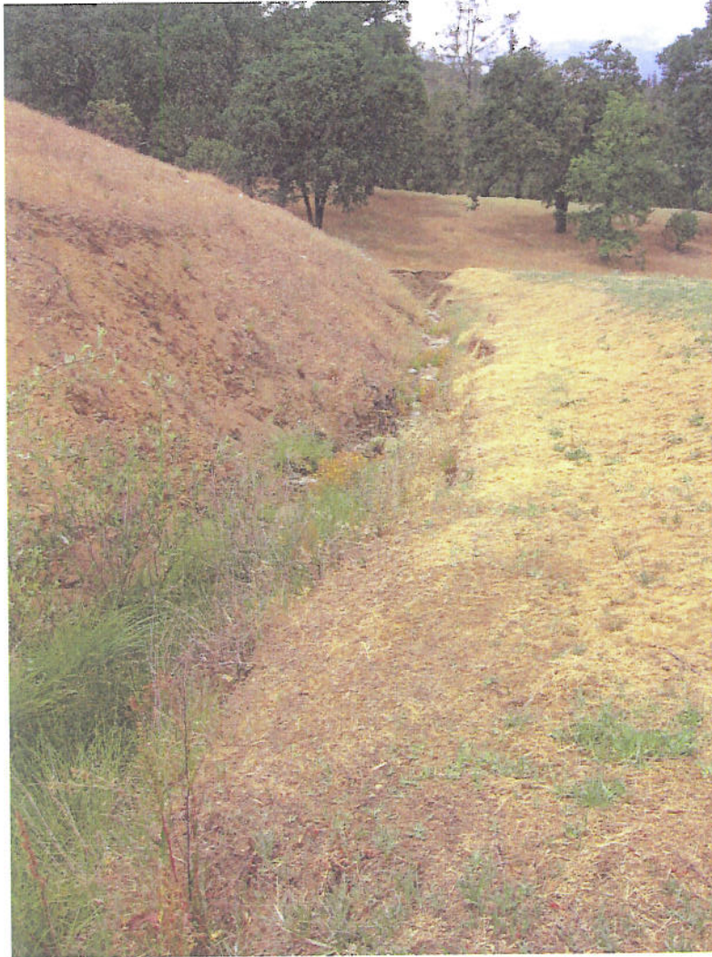
Reservoir named in Permit 18997 Top of spillway looking downstream
