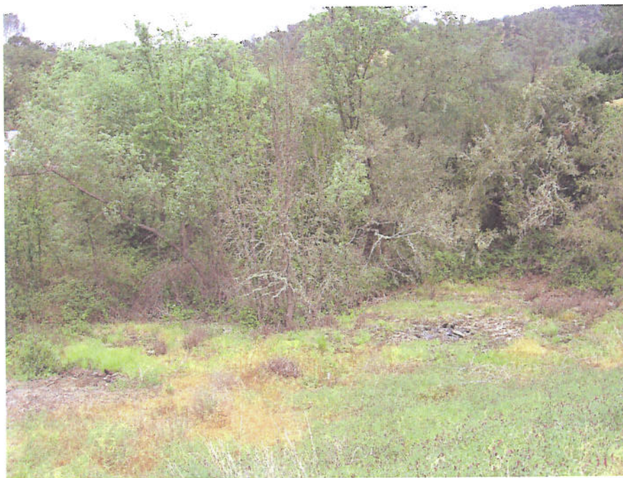
Reservoir named in Permit 18997 Standing on dam looking downstream
