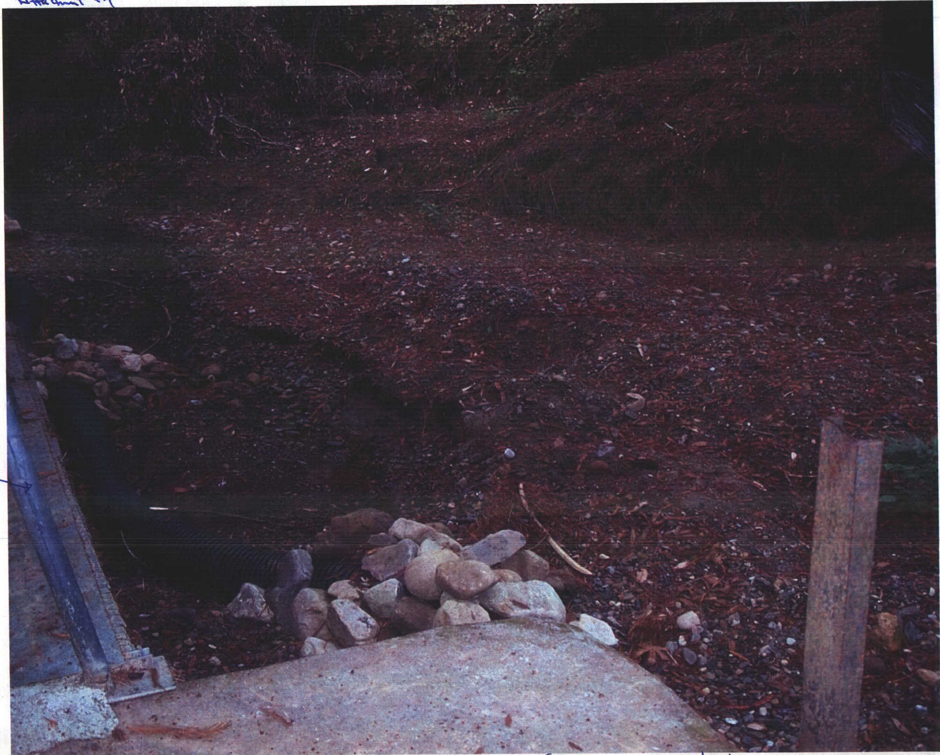
Upstream of Dam
