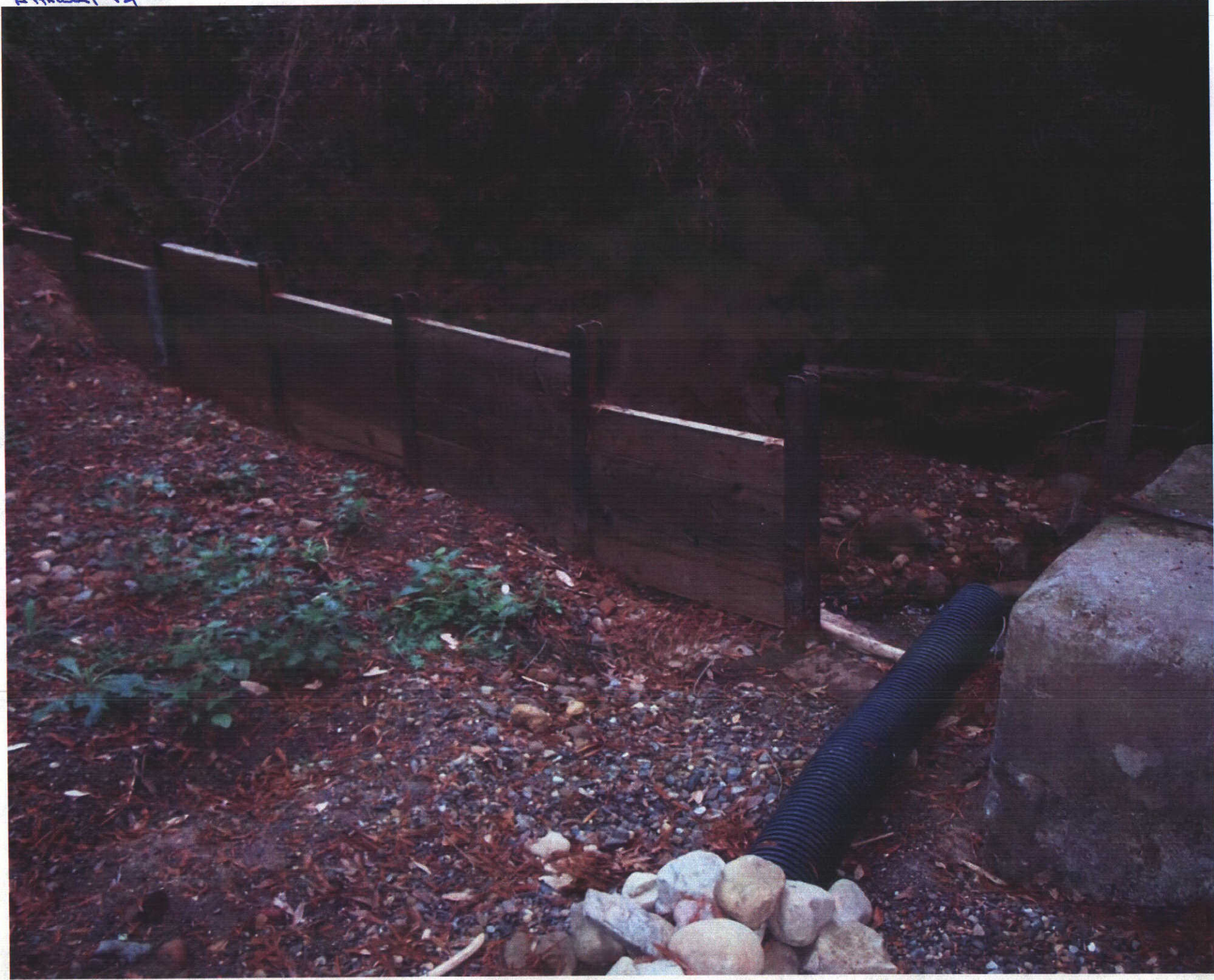
Top of Diversion Dam looking downstream
