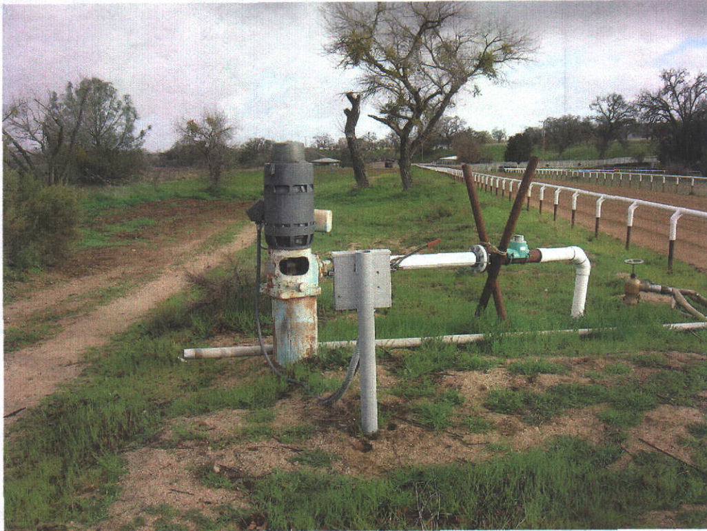
License 7070 - Looking northwest (upstream) from the point of diversion
