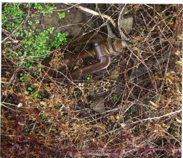
Control Valve of Highline Ditch
