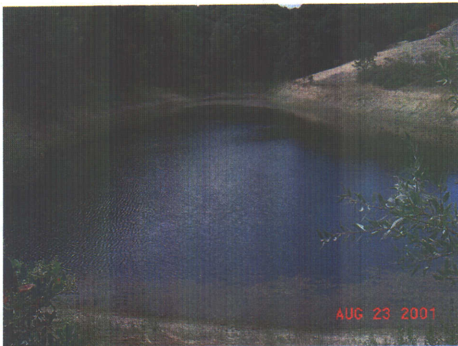
The Middle Reservoir looking north from the dam.
