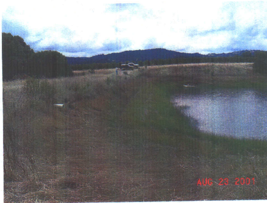
The Upper Reservoir looking west across the dam. Note the spill pipe in the left side of the photograph. The former spillway observed at licensing has been filled.
