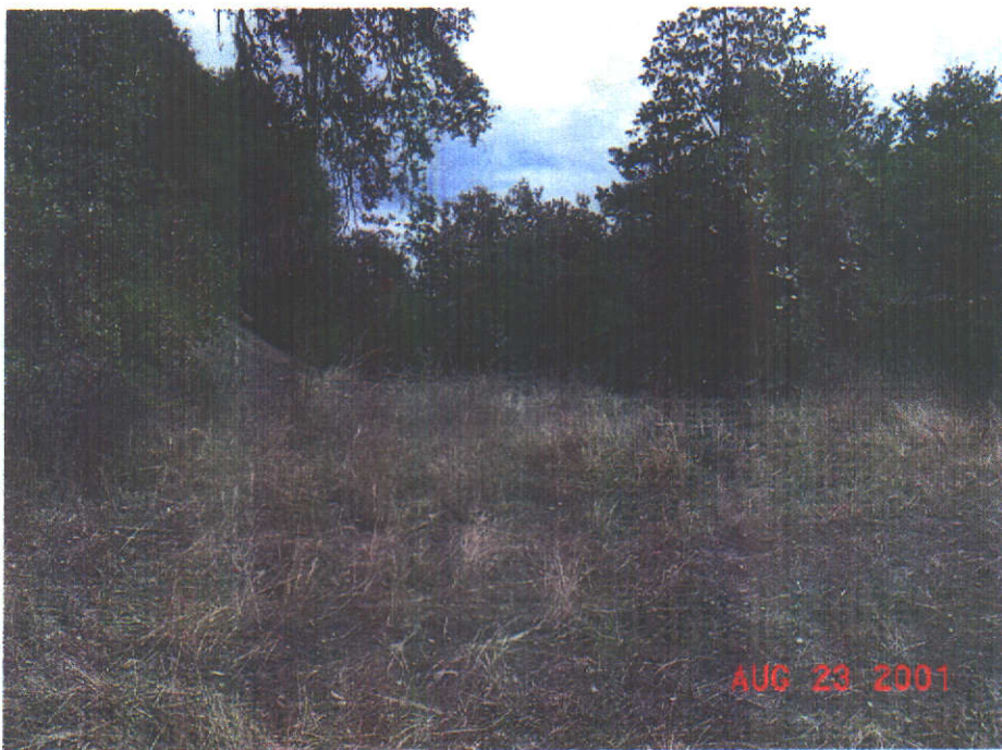
The spillway at the Middle Reservoir looking south.
