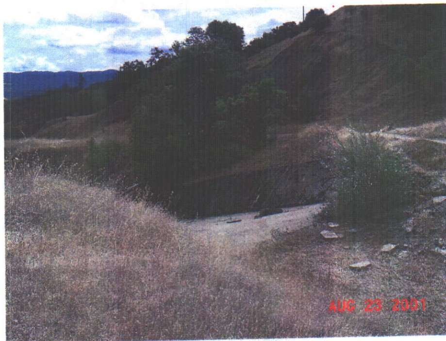
Spillway at Round Mountain Reservoir.
