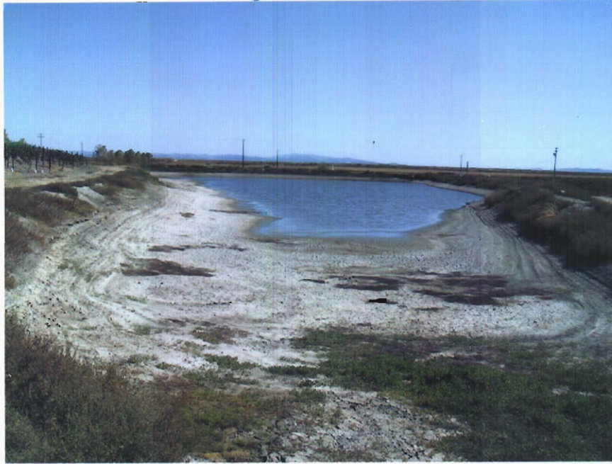
Reservoir No. 2B – Looking Southeast
