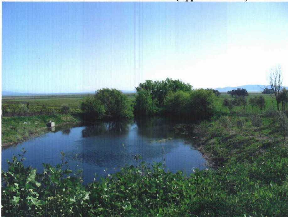
Downstream of Point of Diversion No. 6 (Upper Reservoir)
