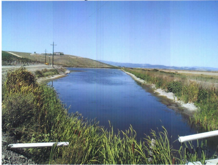
Reservoir No. 5 – Looking Northeast
