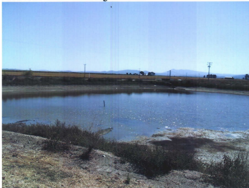
Reservoir No. 2B – Looking South
