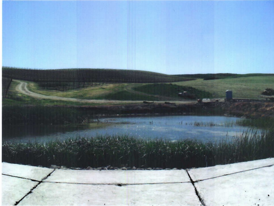
Upstream of Point of Diversion No. 3
