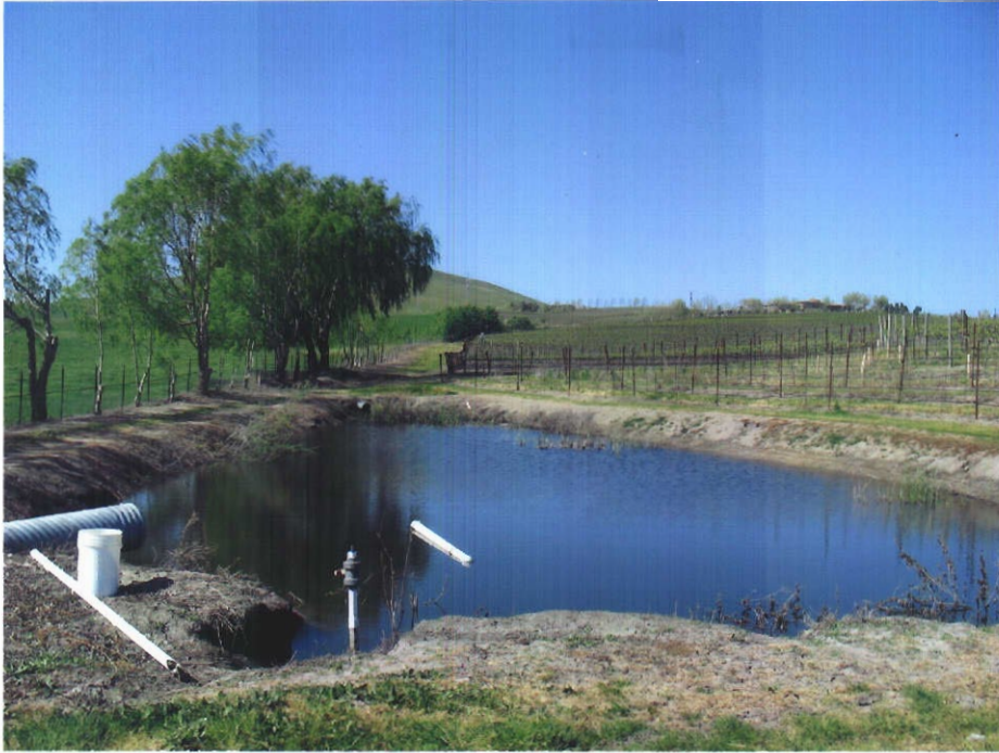
Downstream of Point of Diversion No. 2A
