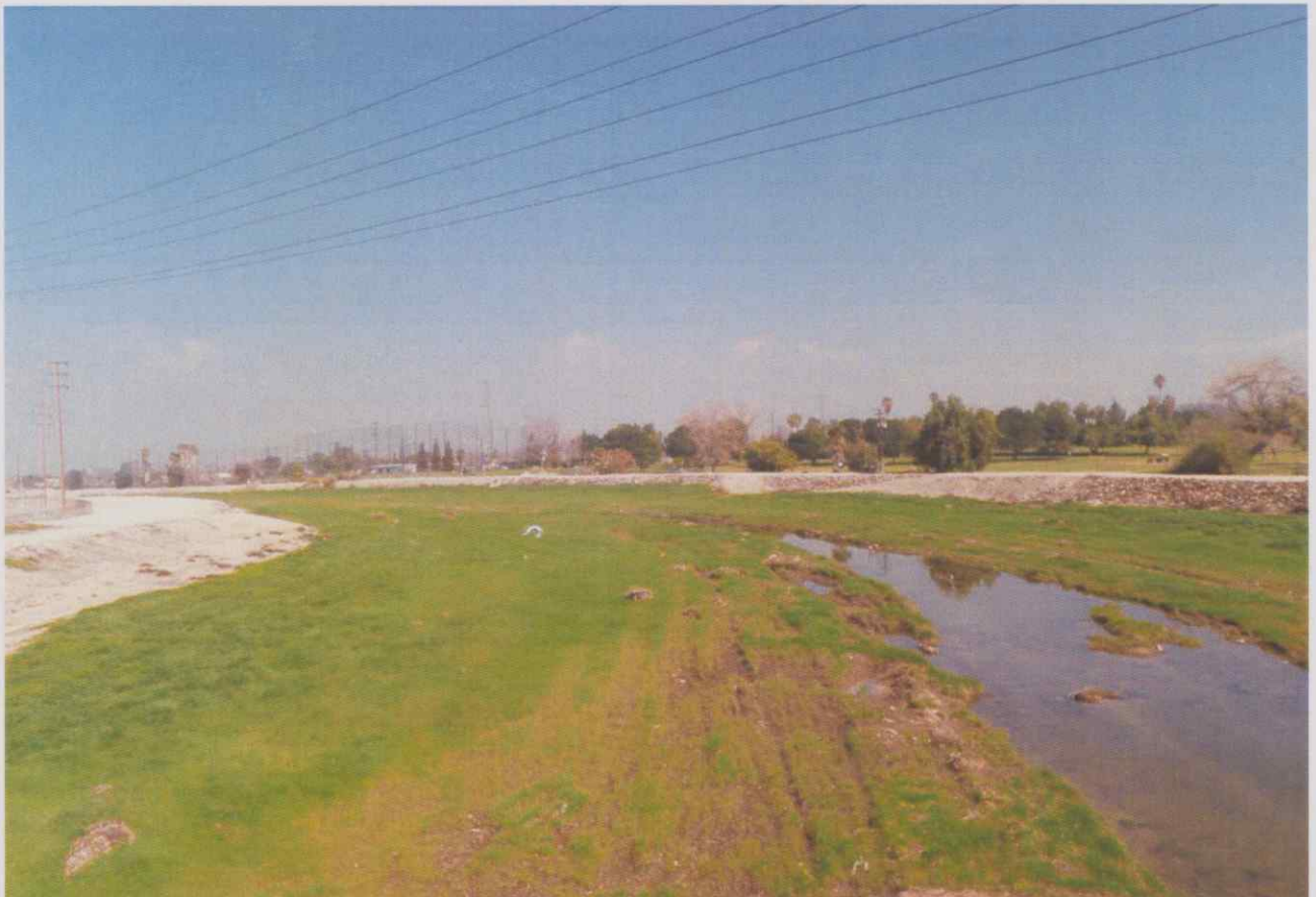
1000-ft Upstream of the SBWRP Outfall, looking North-East.
