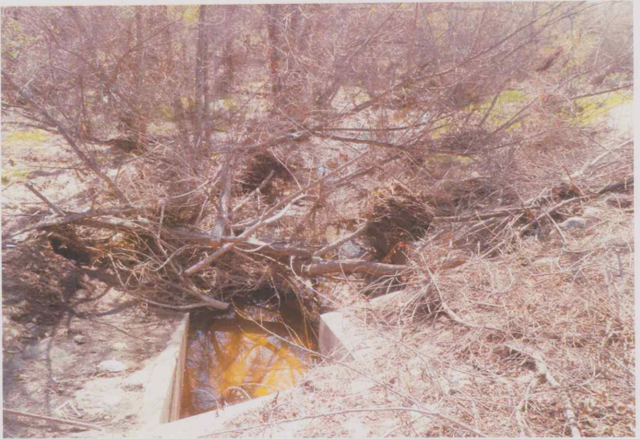
SBWRP Outfall to the Santa Ana River, looking South-West.
