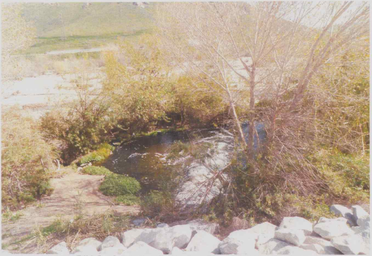
RIX Outfall to the Santa Ana River, looking East.
