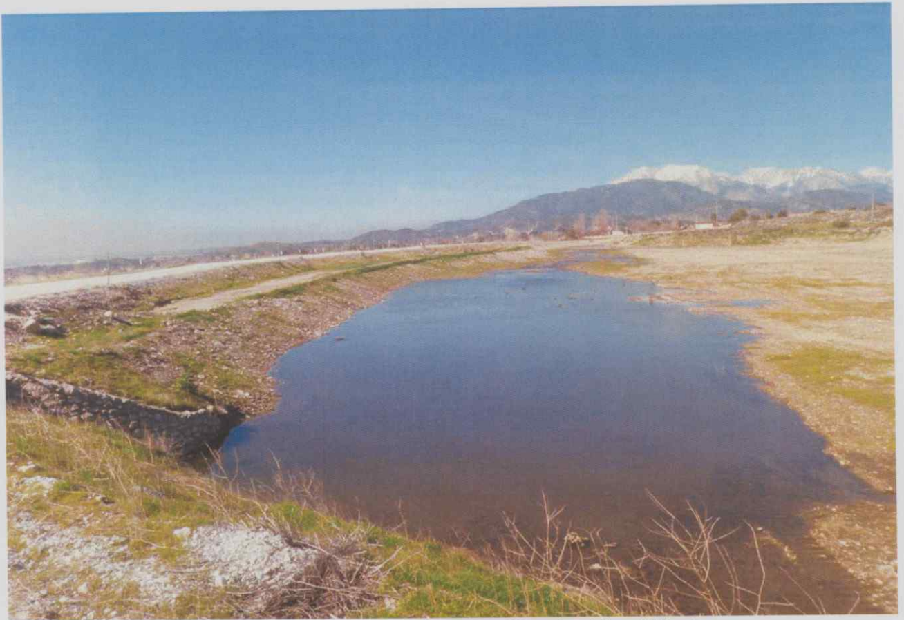
Devil Canyon Recharge Facility, looking West.
