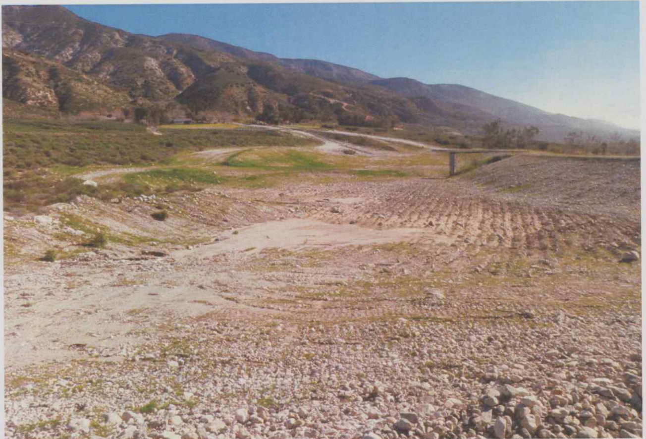
Sweetwater Recharge Facility, looking East.
