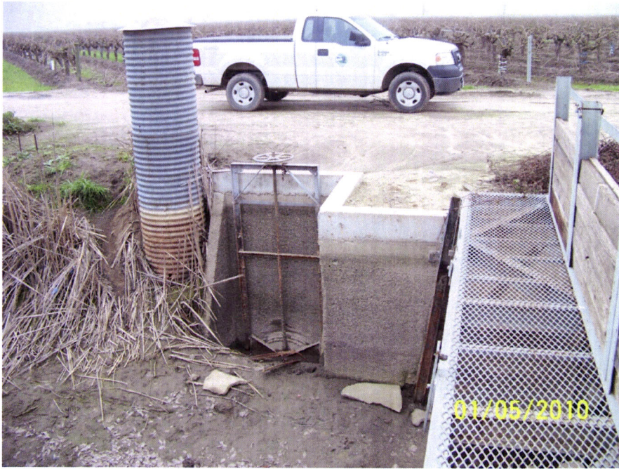
12. South Lateral Diversion Dam Point of Rediversion on Cottonwood Creek
