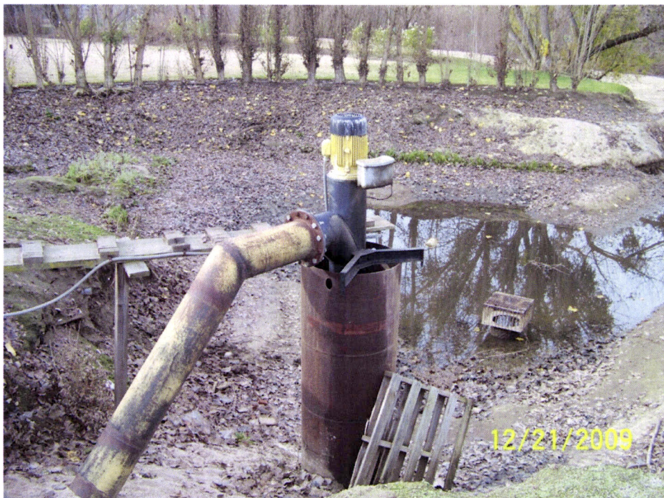
7. Isla Vista Farms LLC Pump Point of Rediversion on Fresno River at River Mile 23.49
