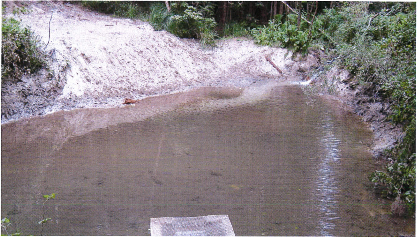
Point of Diversion at Waterfall Gulch from Intake Looking Upstream (July 30, 2013)
