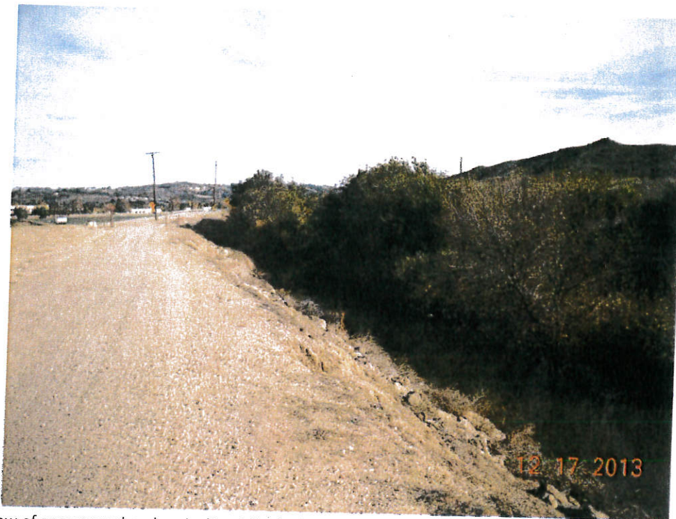
Photo 5. View of access road and agricultural fields along the north bank and riparian zone along the south bank of Conejo Creek upstream of the CWRP. View looking upstream
