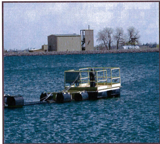
Figure 1-6 Floating Vertical Pumps
