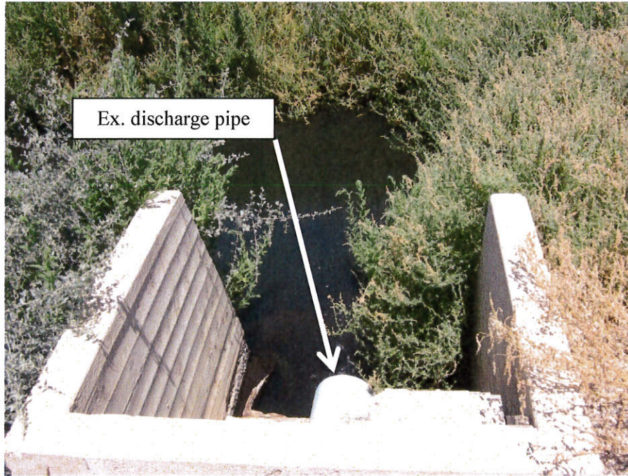
Photo 1: Existing discharge point Date Taken: August 8, 2013
