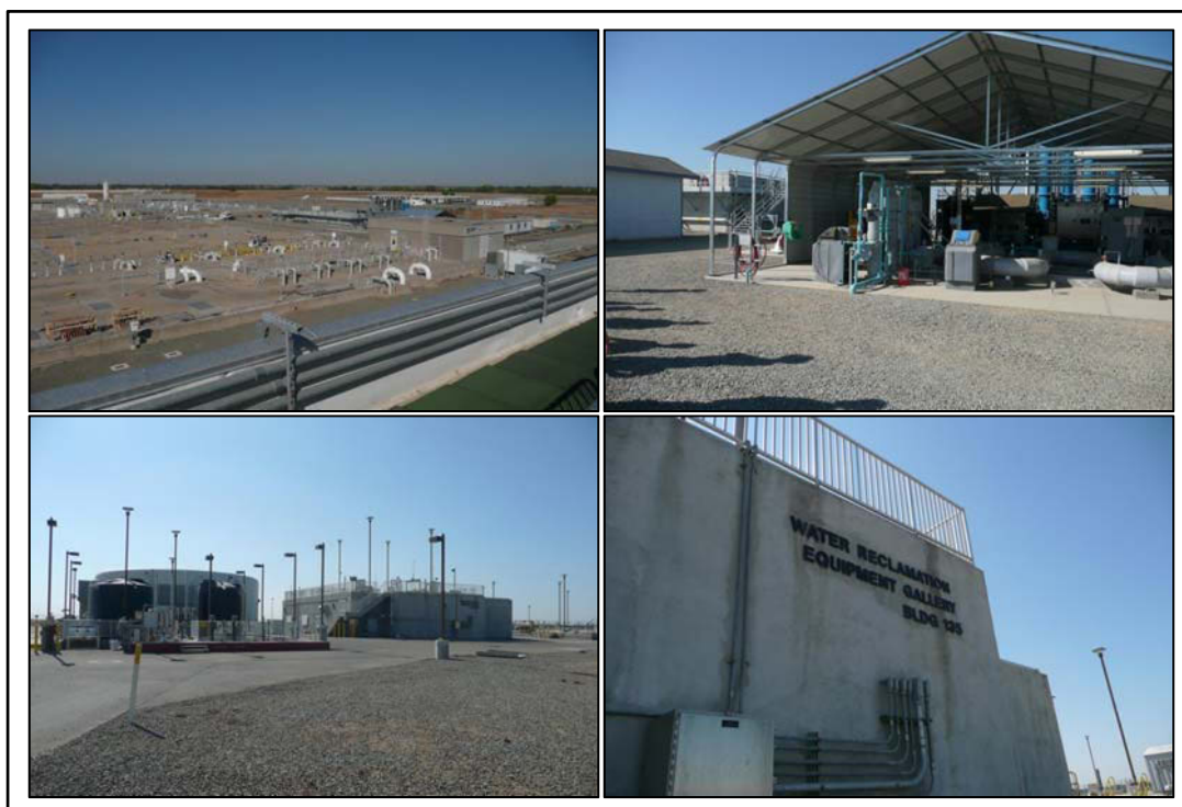
Figure 3.1-2: Existing Facilities at SRWTP
