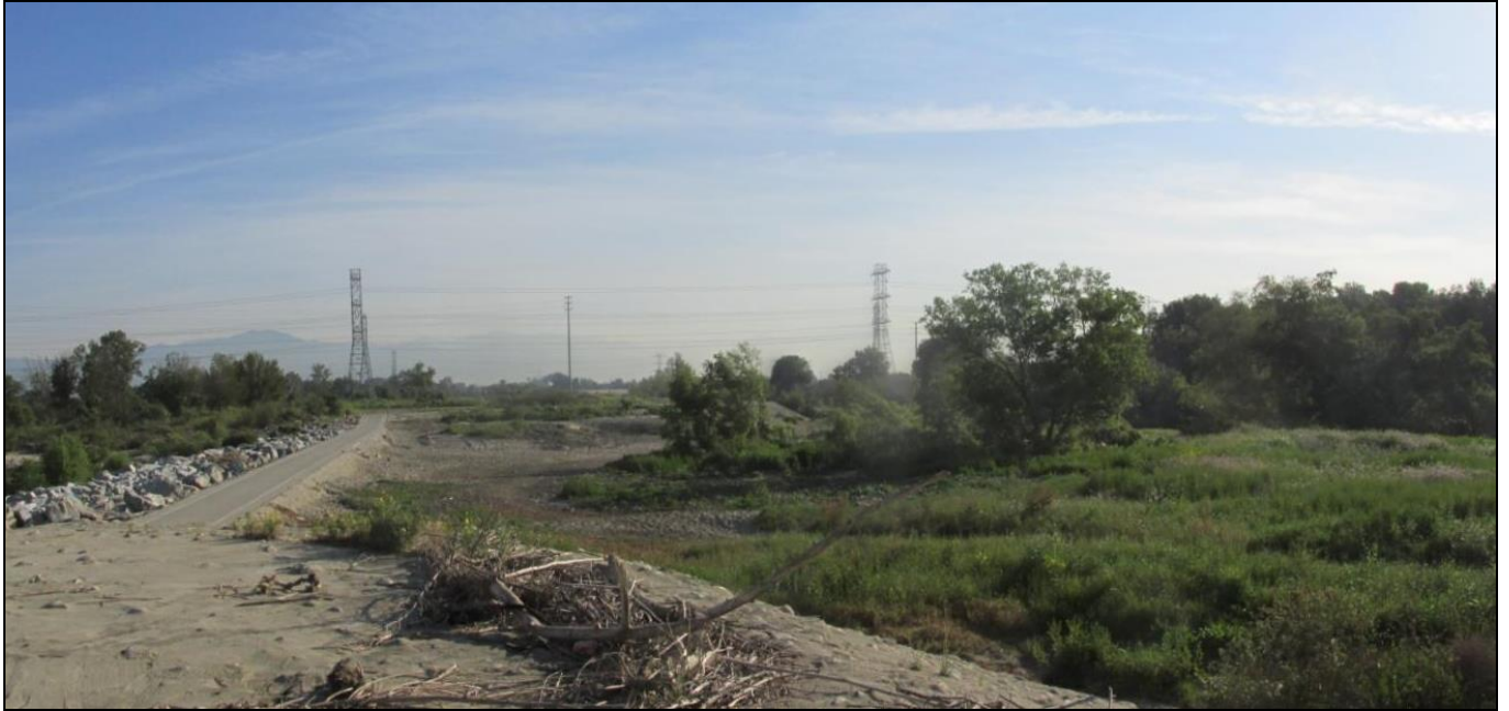
Photo 1: Whittier Narrows (WN) Dam as seen facing north from downstream of the dam.
