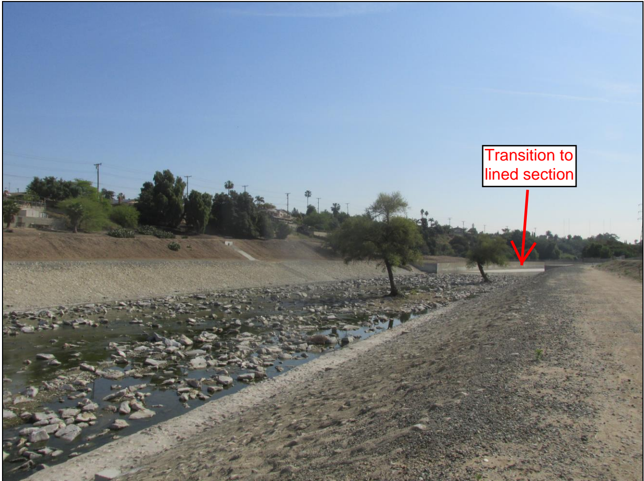
Photo 13: Transition from unlined to lined section of the San Jose Creek.
