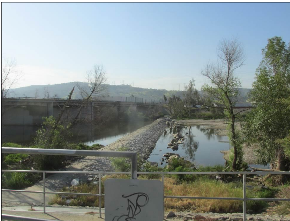
Photo 4: SGR Weir 2 as seen facing east.
