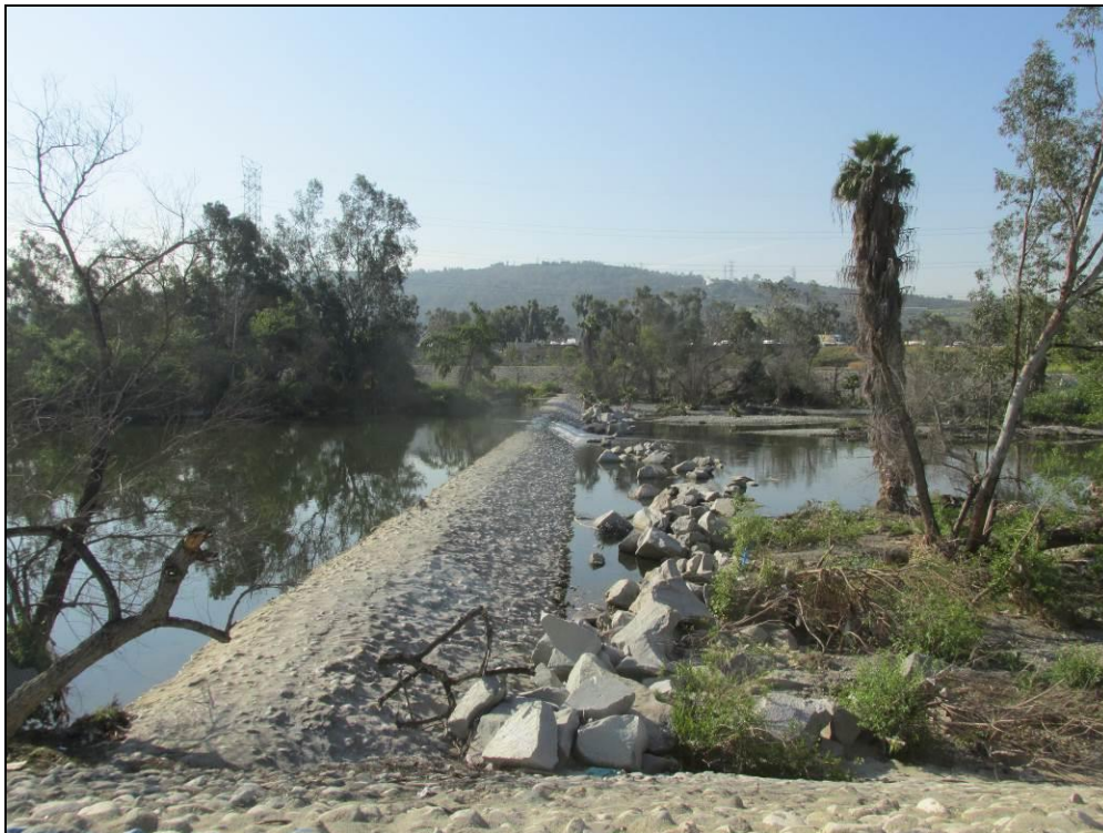
Photo 6: SGR Weir 4 as seen facing south.
