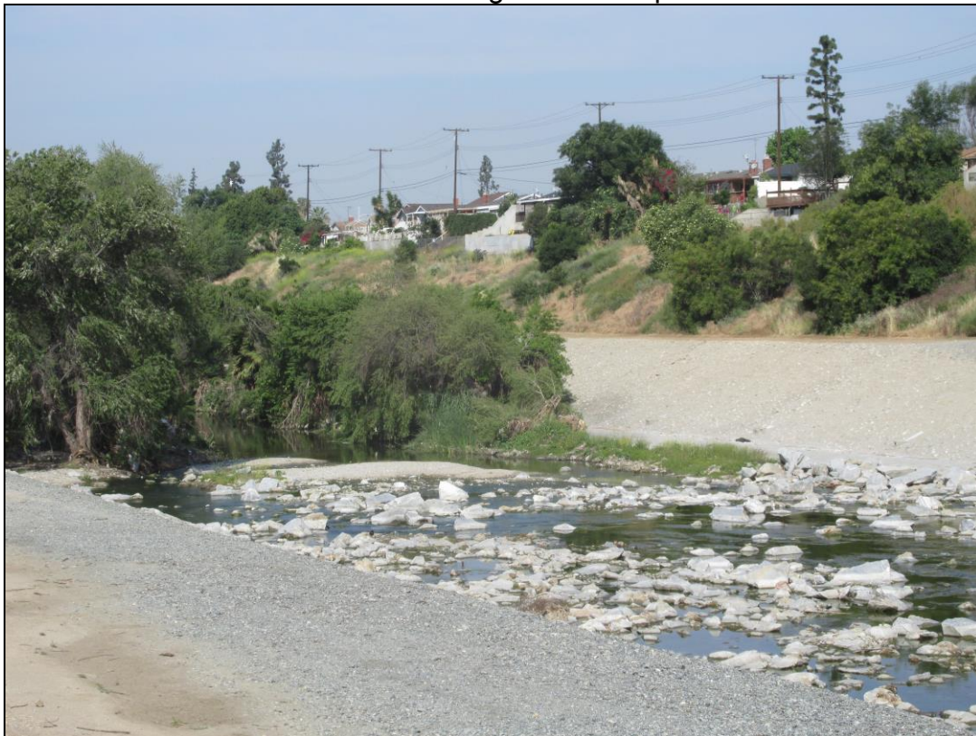
Photo 12: Unlined section of the San Jose Creek.
