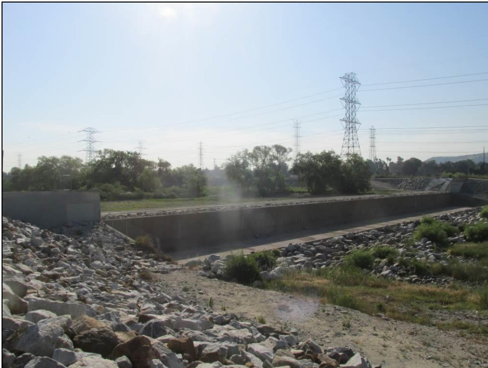
Photo 8: SGR Weir 5 as seen facing east.
