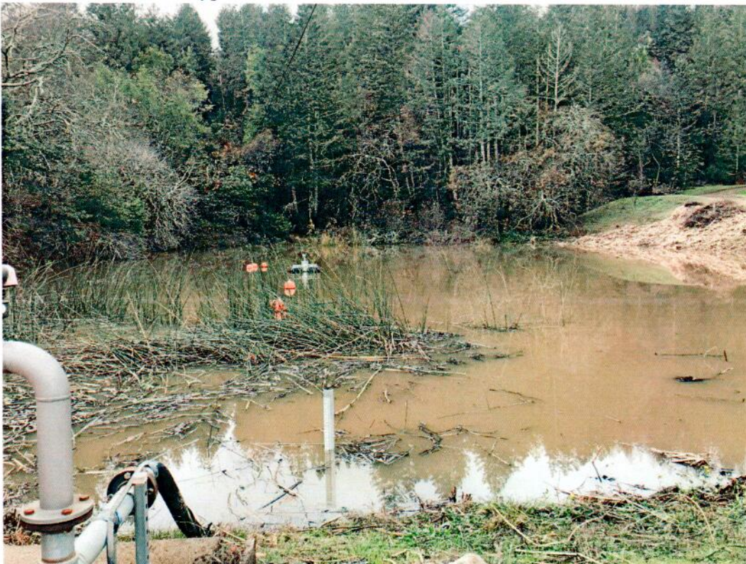
Point of Diversion #1 – On Dam Looking Upstream
