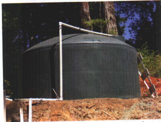
Figure 1: Typical Water Storage Tank w/PVC Line
