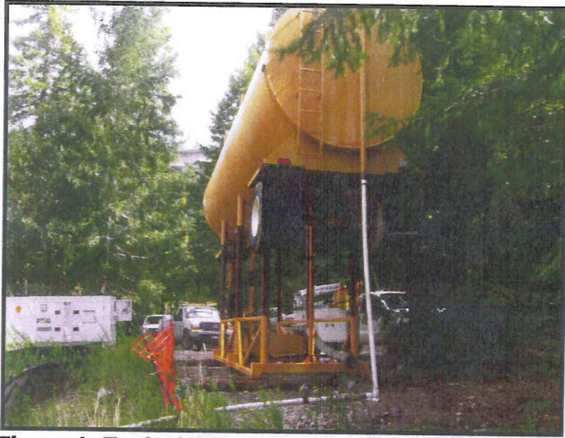
Figure 1: Typical Water Storage Tank w/PVC Line
