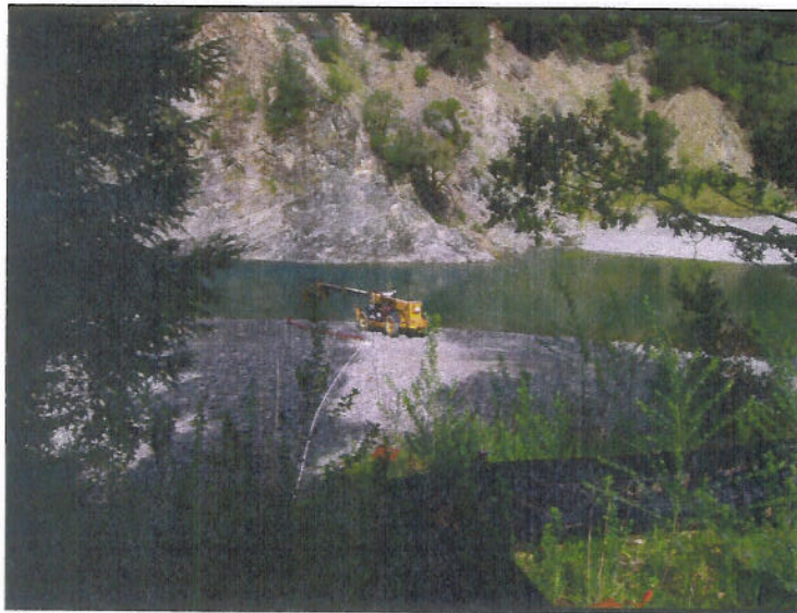
Figure 4: Placement of pump and filter at POD 1
