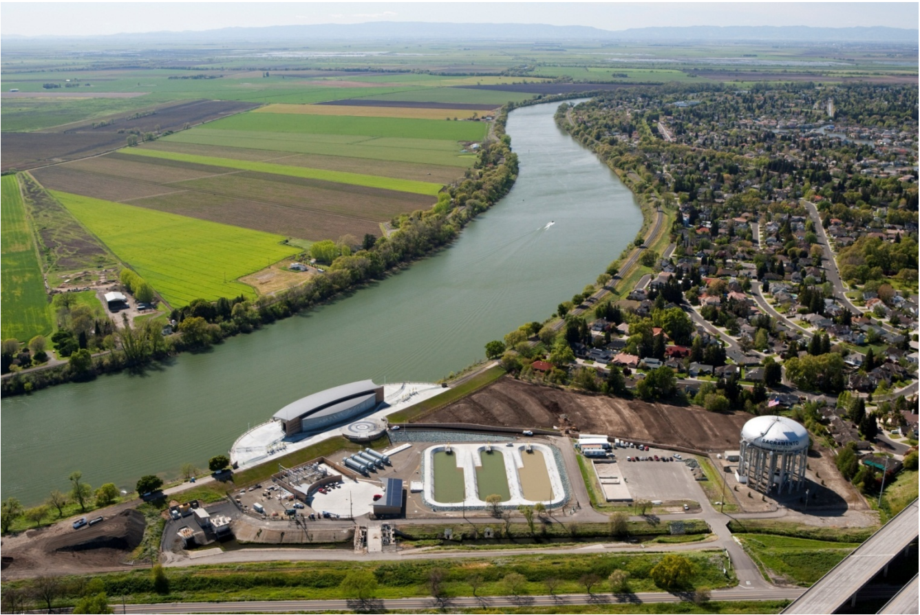
FRWP Intake on the Sacramento River near Freeport
