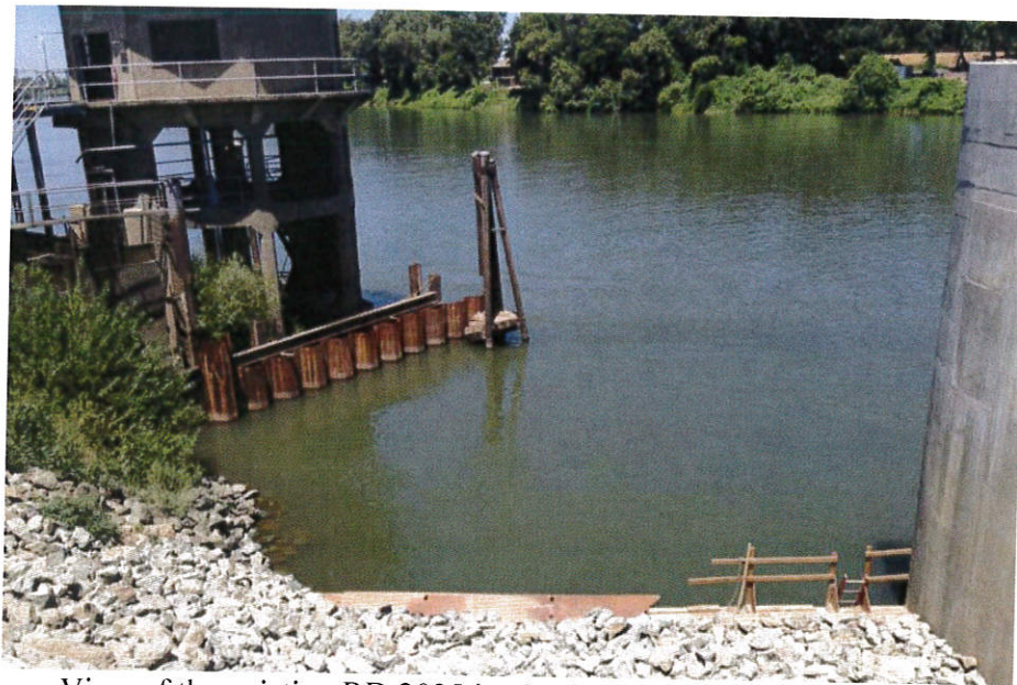
View of the existing RD 2035 intake facing north (upstream) from the joint intake facility (July 12, 2016)
