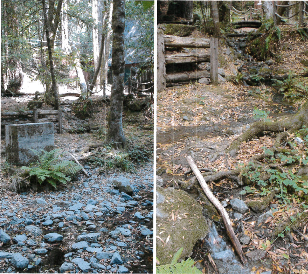
Left: Rock lined channel used to transmit release water to Dutch Bill Creek. (August 18, 2015) Right: Same channel with test release (August 28, 2015)
