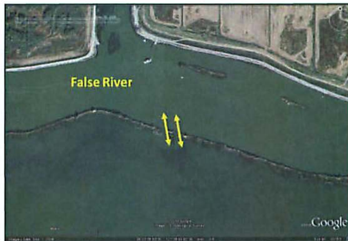
Figure 76. Breaches in an old levee along False River.
