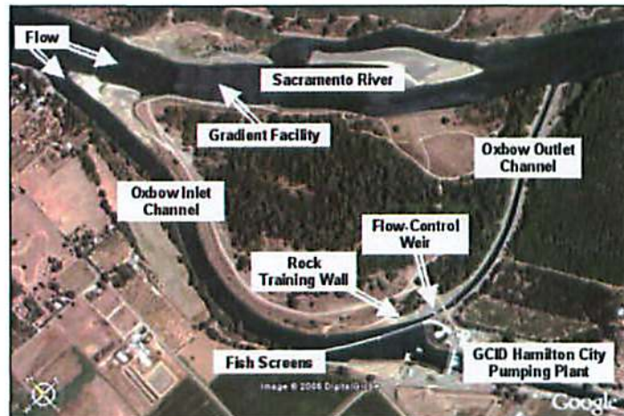
Figure 35. Aerial view of the new GCID fish screens and gradient facility on the Sacramento River near Hamilton City (from Vogel 2008a).
