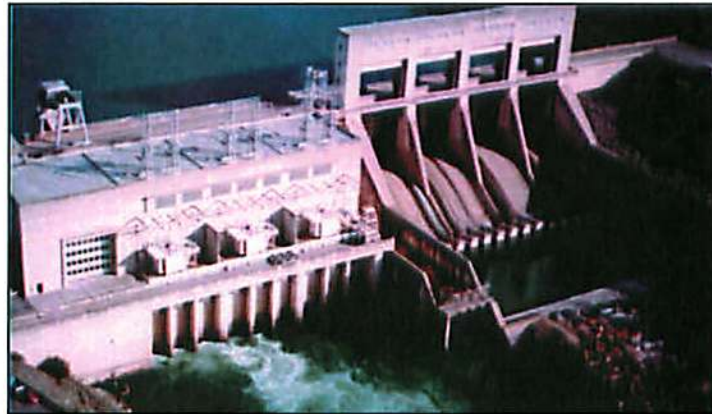
Figure 13. Keswick Dam located at river mile 302 on the upper Sacramento River. The stilling basin on the right side of the picture used to trap adult anadromous salmonids. Aerial photo by Dave Vogel.
