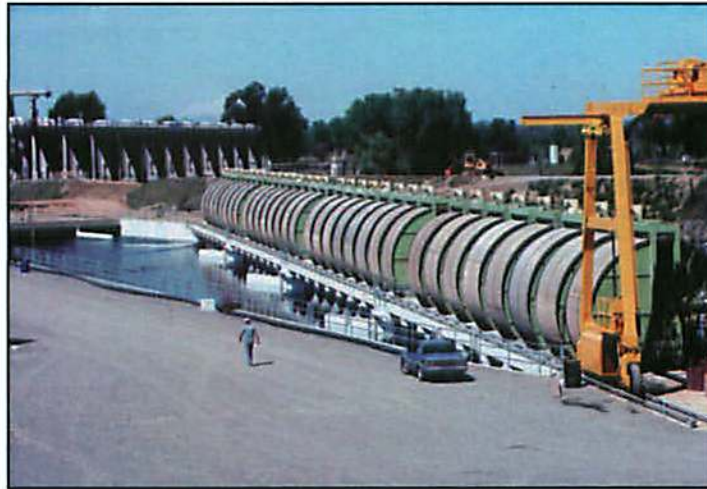
Figure 36. State-of-the-art angled rotary drum screens installed at the headworks to the Tehama-Colusa Canal and Corning Canal at RBDD in 1990. Photo by Dave Vogel.
