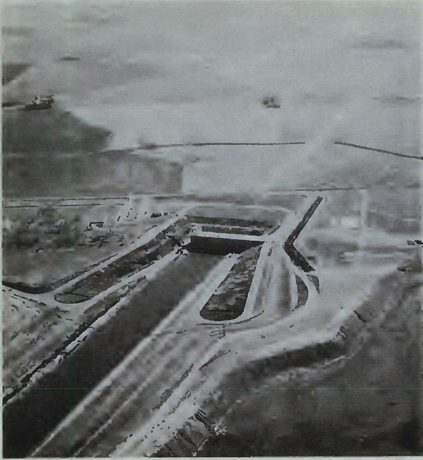
Tracy Pumping Plant
