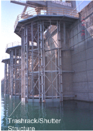
Figure 12. Powerhouse Intakes – Top of Shutters Showing.
