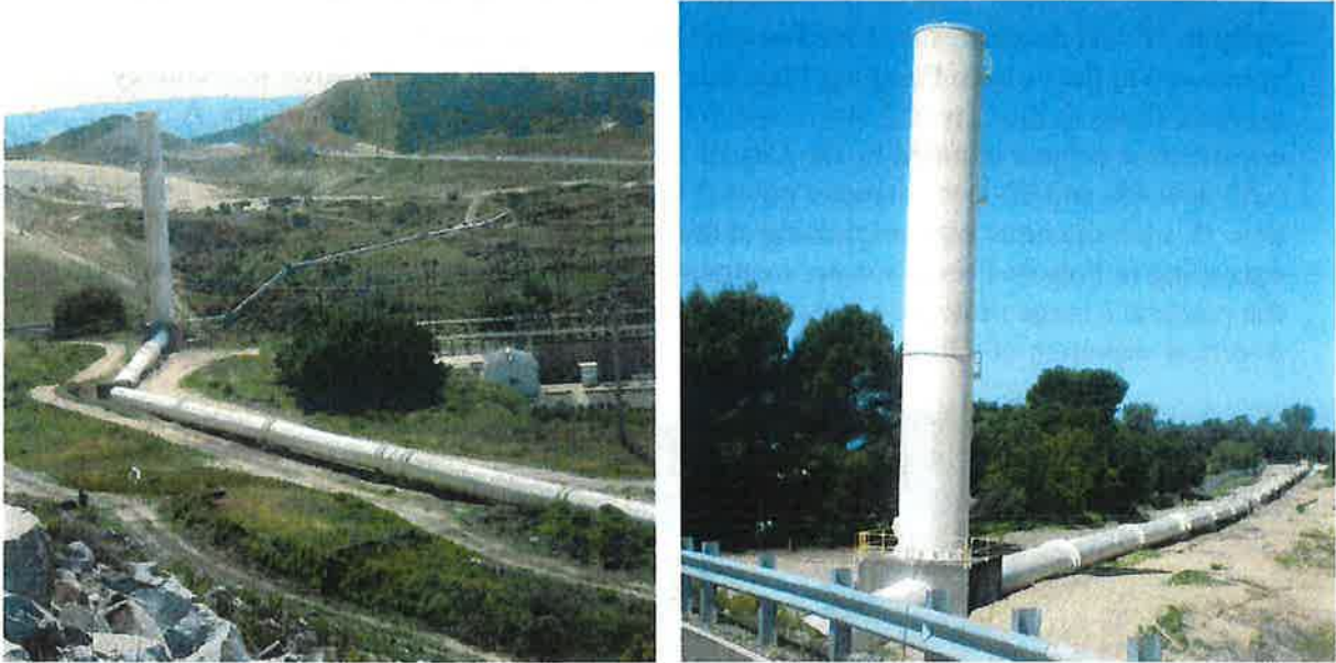
Figure 2-4 North Fork Pipeline and Main Standpipe, Looking East (Picture on Left, with “Old” [2009] Natoma Pipeline in Background), and 84-inch North Fork Pipeline and 10-foot-diameter Standpipe, Looking West Toward Hinkle Y (Picture on Right)
