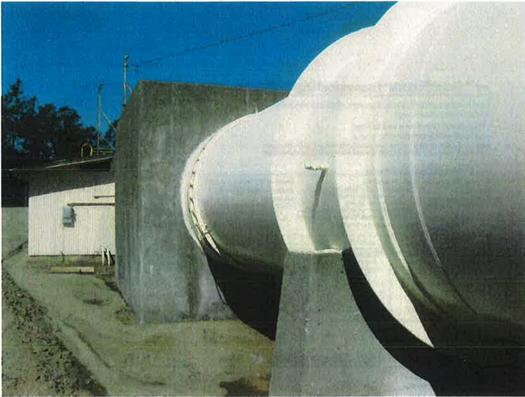
Figure 3. Pressure Gage Location at Hinkle Y
