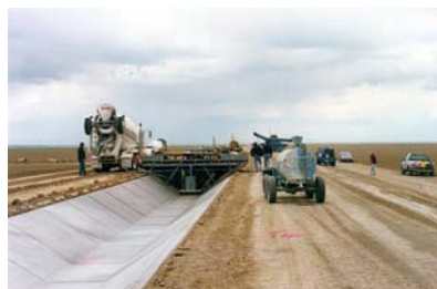
Canal Lining to Prevent Seepage Losses
