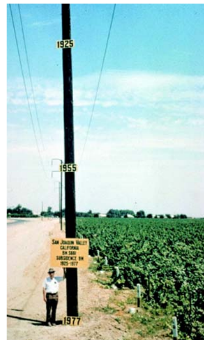
FIGURE 2-10 Land Subsidence Recorded on a Telephone Pole in the Central Valley (Source: USGS)
