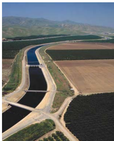
Statewide water management systems include physical facilities like the California Aqueduct. (Source: DWR)
