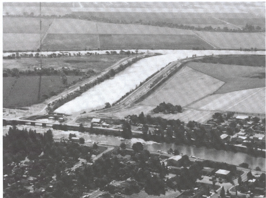
The Delta Cross Channel, constructed by the Bureau of Reclamation in 1951, connects the Sacramento River (foreground) with Snodgrass Slough and the Mokelumne River system.
