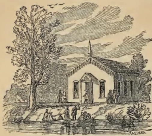
CHURCH ON THE RIVER, NINE MILES ABOVE STEAMBOAT SLOUGH.
