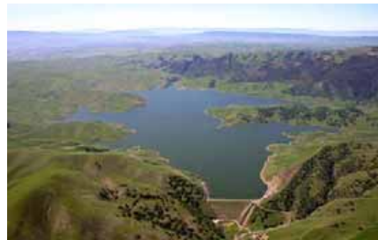
CCWD’s 100,000 AF Los Vaqueros Reservoir near Byron improves water quality and emergency water supply reliability for CCWD customers. The reservoir is typically filled in the spring and early summer when Delta water quality is good, and used to blend with Delta water in the fall when Delta water quality is typically poor. (Photo by Stephen Joseph)
