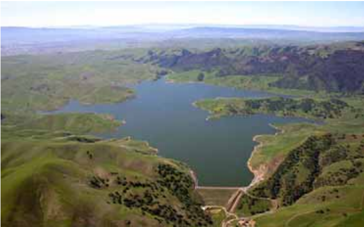
Expansion of Los Vaqueros Reservoir in Contra Costa County could improve the quality of water supplies delivered to Bay Area agencies from the Delta.
