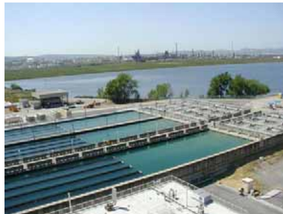
Sedimentation basins at CCWD's Bollman Water Treatment Plant. Shown in background is Mallard Reservoir, the 3,000 acre-feet forebay for the drinking water treatment plant.
