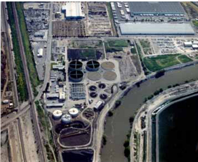
The City of Stockton's 48-million-gallon per-day Regional Wastewater Control Facility, located beside the San Joaquin River just north of Highway 4.
