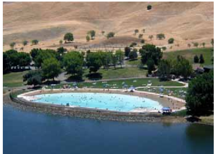
The swimming lagoon at Contra Loma Reservoir was completed in spring 2002. The almost one-acre lagoon protects public health by eliminating body contact with CCWD's drinking water supply stored in the 2,500 acre-foot Contra Loma Reservoir in Antioch.
