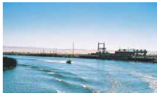
Looking southwestward at CCWD'S Old River at Highway 4 intake, completed in 1997.
