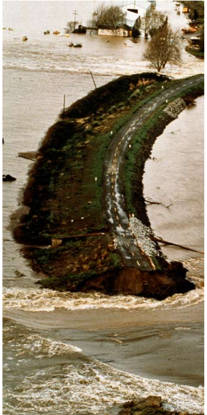
Levee breaches at Tyler Island [1986]. Source: DWR
