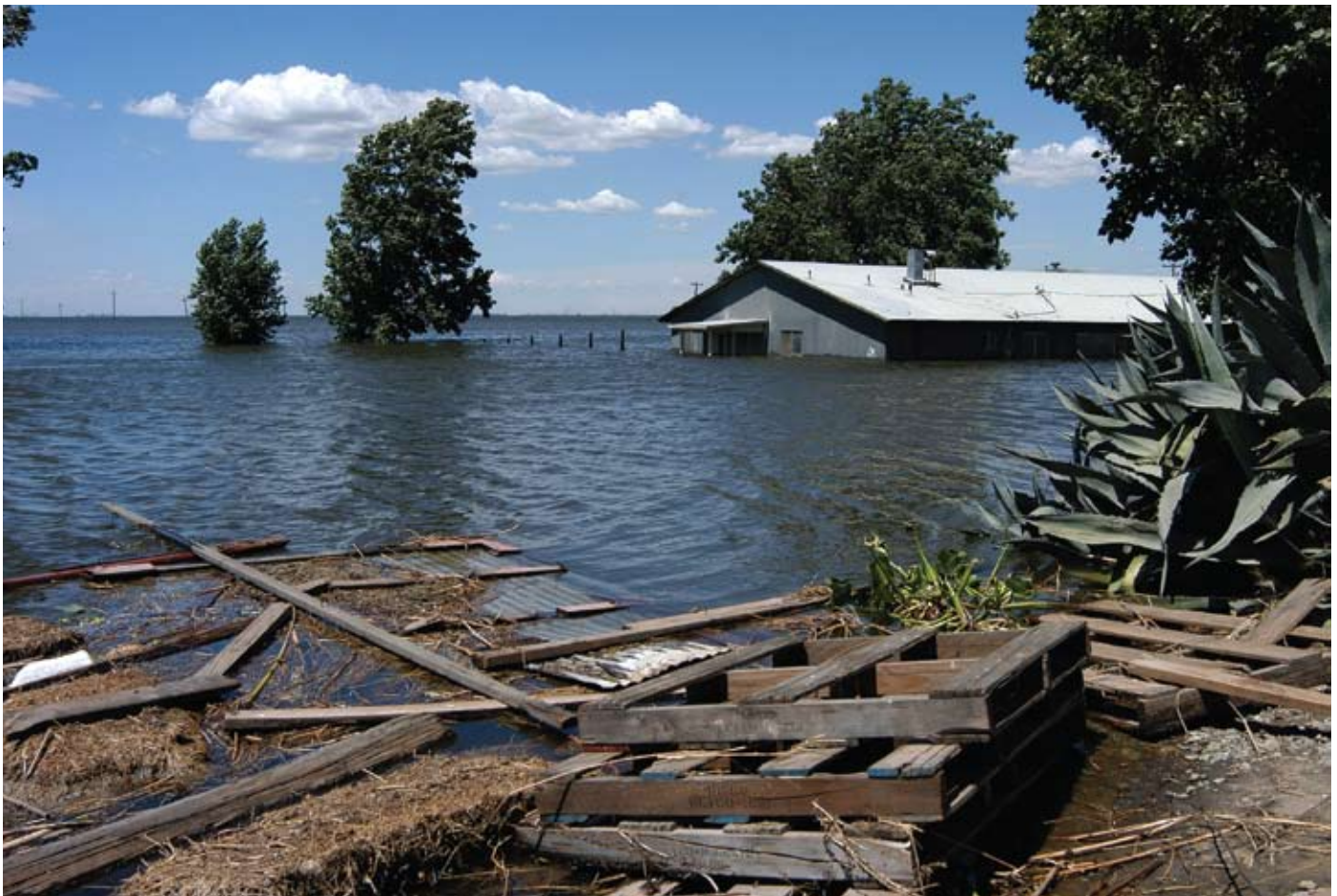
Flood damage – Delta [June 7, 2004]. Source: DWR
