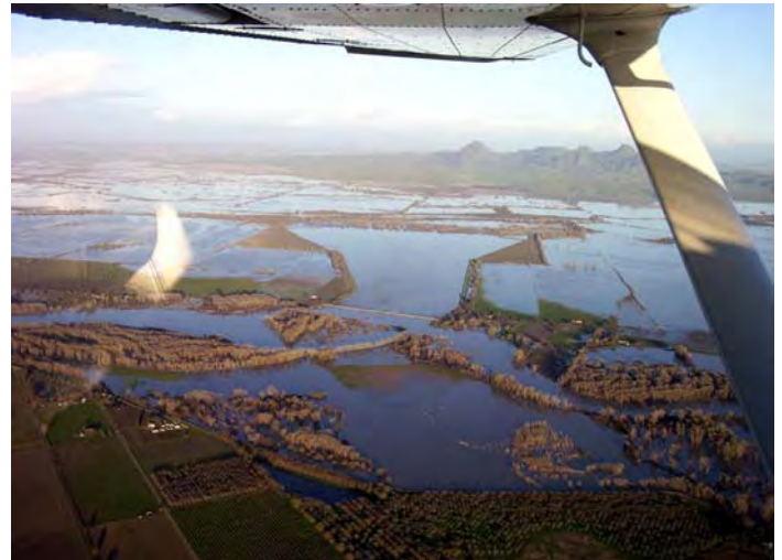
Figure 4, Colusa Weir, January 1997
