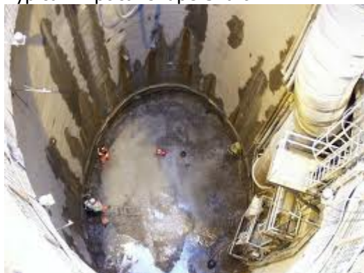
Typical Elliptical-shape Shaft
