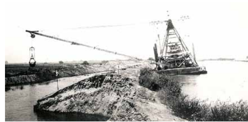
Figure 4.14. Dredge building levee showing side-ditch. This early 1900s photograph shows a sidedraft clamshell dredge working on a levee, drawing material from a ditch. Over the past century, many of these ditches have become a part of the main channel. (Covello ca. 1900, courtesy of Bank of Stockton Historical Photograph Collection)
