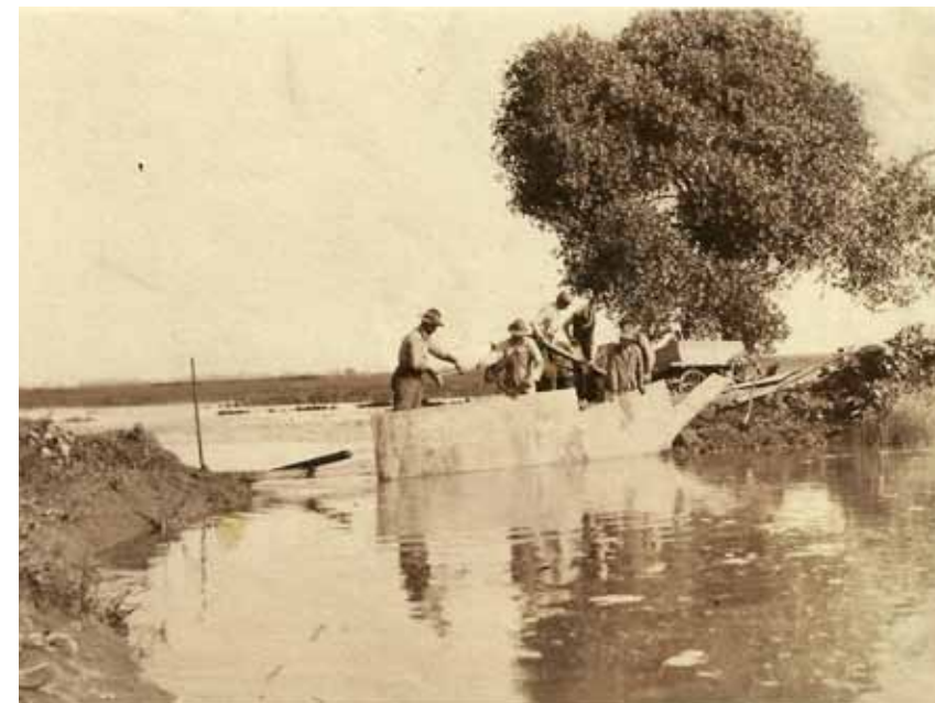
Figure 1.12. Damming sloughs. In the early years of reclamation, most of the smaller sloughs that brought tides to the interior of Delta islands were dammed either with tide gates or by building a levee across them. (Unknown ca. 1900, MS 229, Dyer Photograph Album, courtesy of Holt-Atherton Special Collections, University of the Pacific Library)
