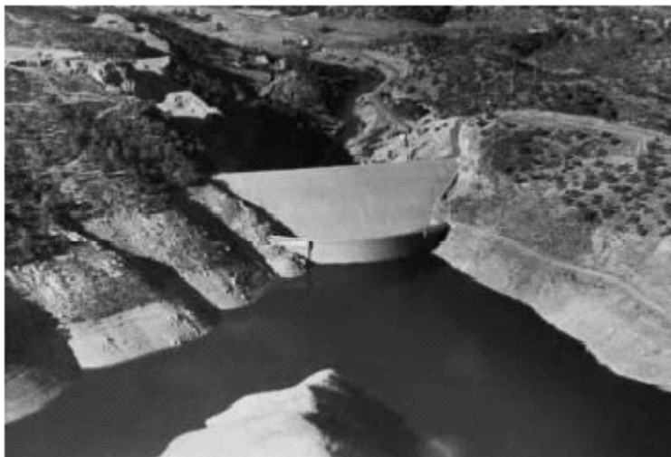
Figure 5.6. The Old Exchequer Dam is curved and shown in front of the New Exchequer Dam (Source: http://www.mercedid.org/_images/water_maincanal_sep02.pdf ).
