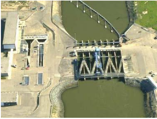
The SWP's Skinner Fish Protection Facility
