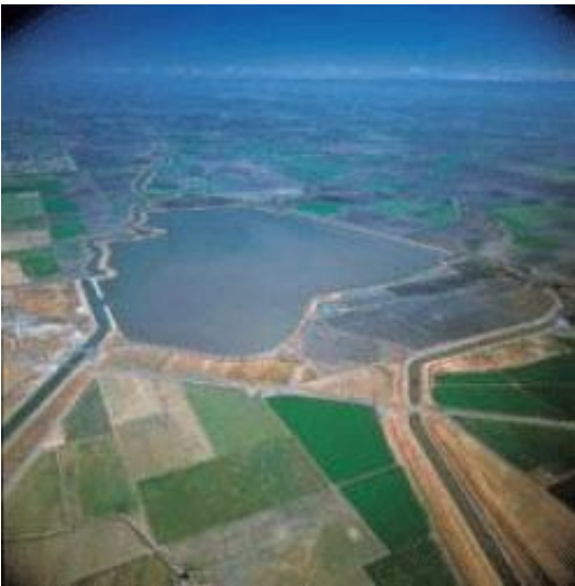
Aerial view of Clifton Court Forebay
