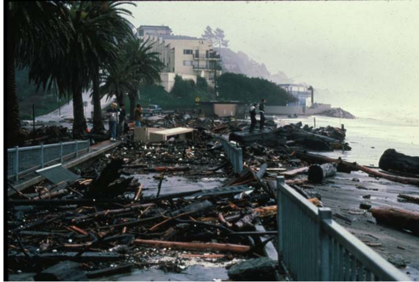
FIGURE 5.12 Rio Del Mar on northern Monterey Bay was damaged during the El Niño winter of 1983 by large waves arriving simultaneously with high tides and elevated sea levels. SOURCE: Courtesy of Gary Griggs, University of California, Santa Cruz.
