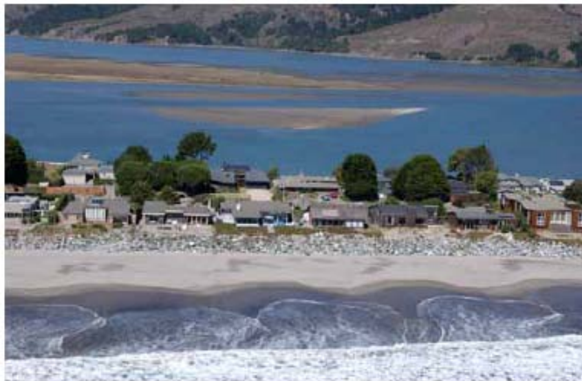
FIGURE 6.7 Developed sand spit at Stinson Beach in Marin County, California, where a revetment has been constructed in an effort to protect the homes. This spit cannot migrate with sea-level rise. SOURCE: Copyright 2002-2012 Kenneth & Gabrielle Adelman, California Coastal Records Project, < www.Californiacoastline.org >.
