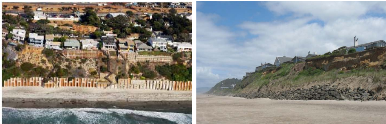
FIGURE 6.4 Seawalls and revetments fronting coastal cliffs and bluffs in California and Oregon. (Left) Concrete and timber seawalls protecting cliff top homes in Solana Beach, California. SOURCE: Copyright 2002-2012 Kenneth & Gabrielle Adelman, California Coastal Records Project, < www.Californiacoastline.org >. (Right) Rip rap protecting bluff top housing along the central Oregon coast. SOURCE: Courtesy of Gary Griggs, University of California, Santa Cruz.
