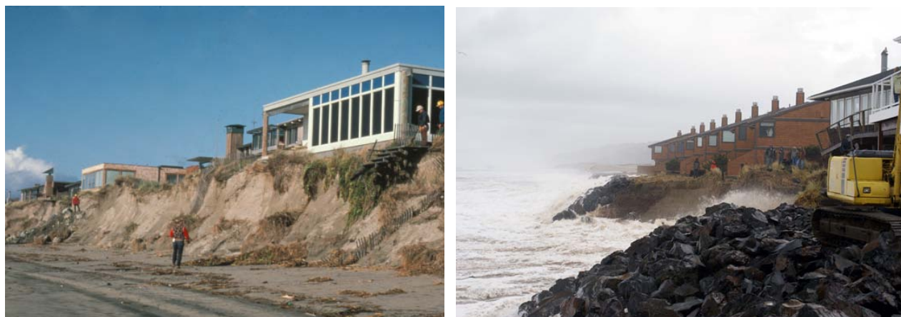
FIGURE 6.9 Construction of private homes on the frontal dunes. (Left) Homes in central Monterey Bay were threatened by erosion during the high tides, elevated sea levels, and large storm wave of the 1983 El Niño. SOURCE: Courtesy of Gary Griggs, University of California, Santa Cruz. (Right) Placement of riprap during storm conditions to protect development on dunes in Neskowin, Oregon. SOURCE: Courtesy of Armand Thibault.
