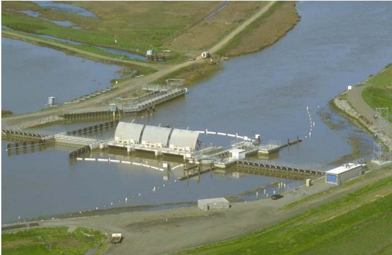
Figure 18. Suisun Marsh Salinity Control Gates. (Source: V. Pacheco.)
