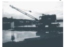
A dredger clears a creek crossing.
