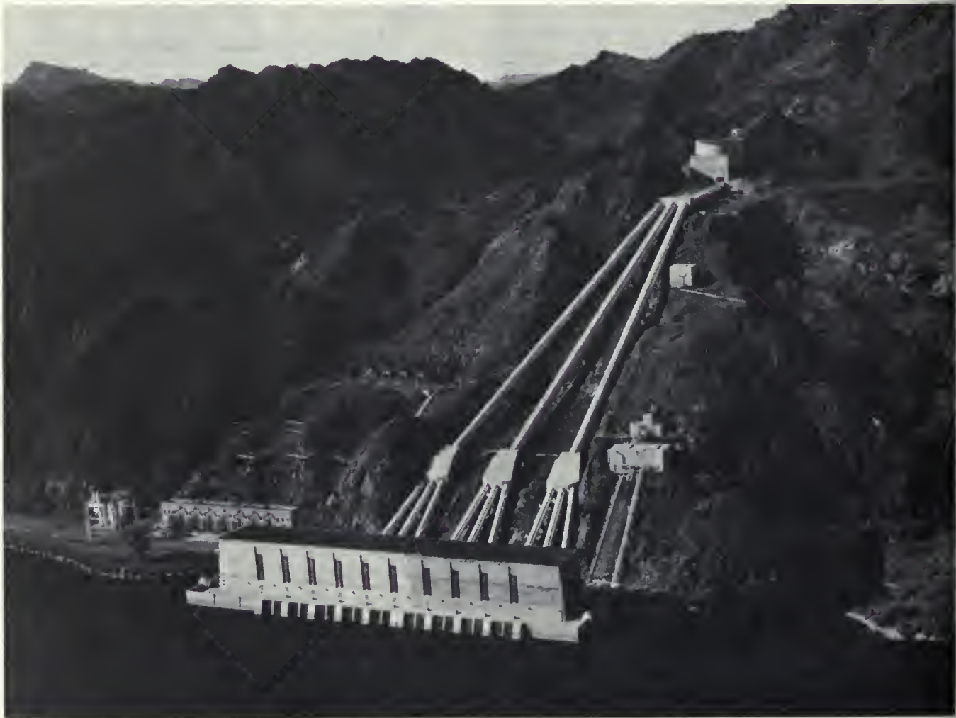
Whitsett Intake pumping plant, a facility of the Colorado River Aqueduct, at Lake Havasu.
