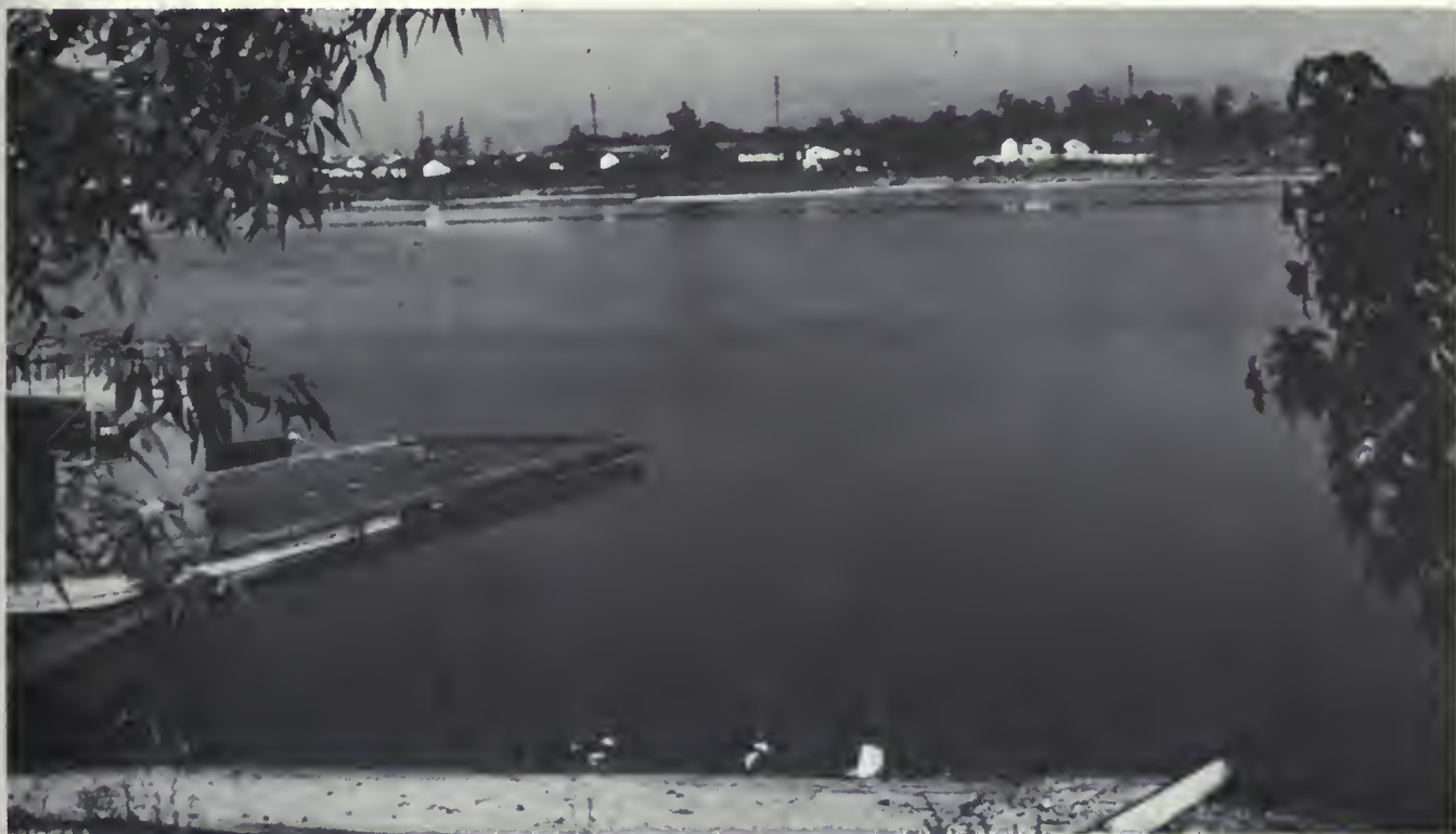
Ground water recharge at Anaheim Lake in Orange County.
