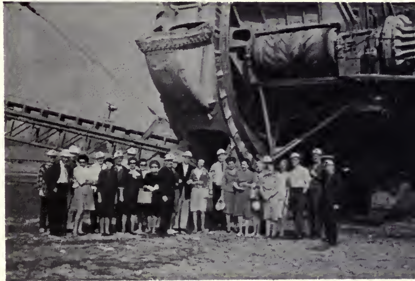
Fifth Annual Inspection of the work at Oroville Dam. Director of the Department of Water Resources, principle staff and their wives, standing near "the monster." March 27, 1966.
