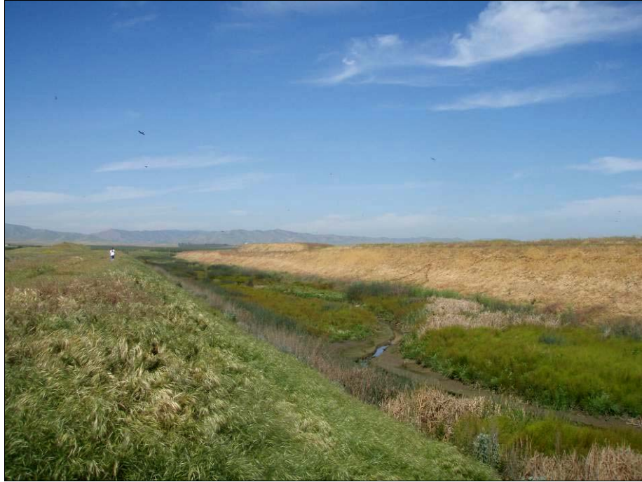
Photograph 2.2.4-6. View of the Unlined Newman Wasteway Where the Wetland Vegetation Approximately 60 feet Across Is Visible
