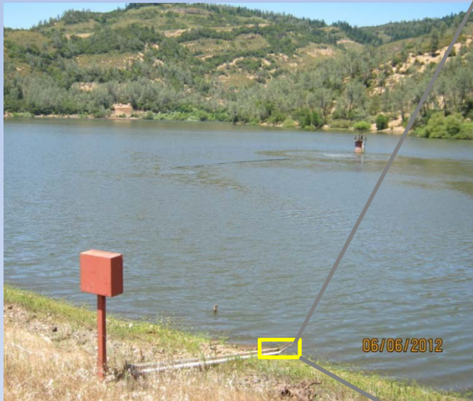
Sloped Staff Gauge
