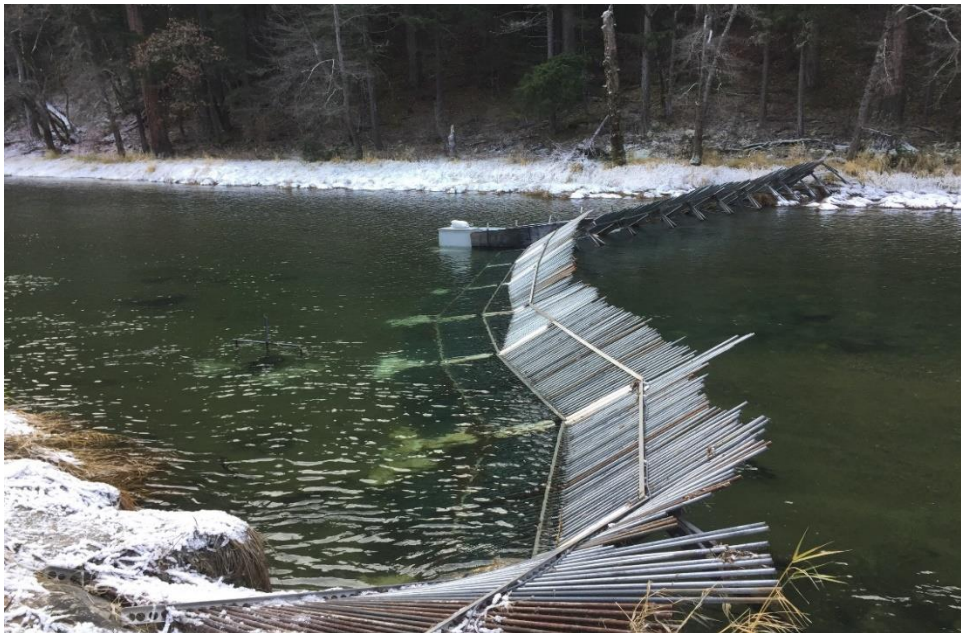
Scott River Fish Counting Facility
