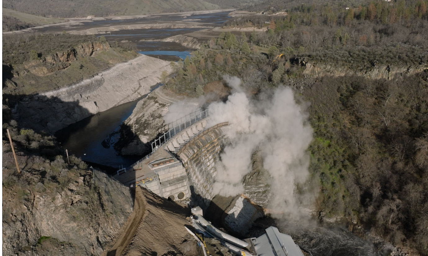
Demolition of Copco 1. Photo credit: Shane Anderson of Swiftwater Films
