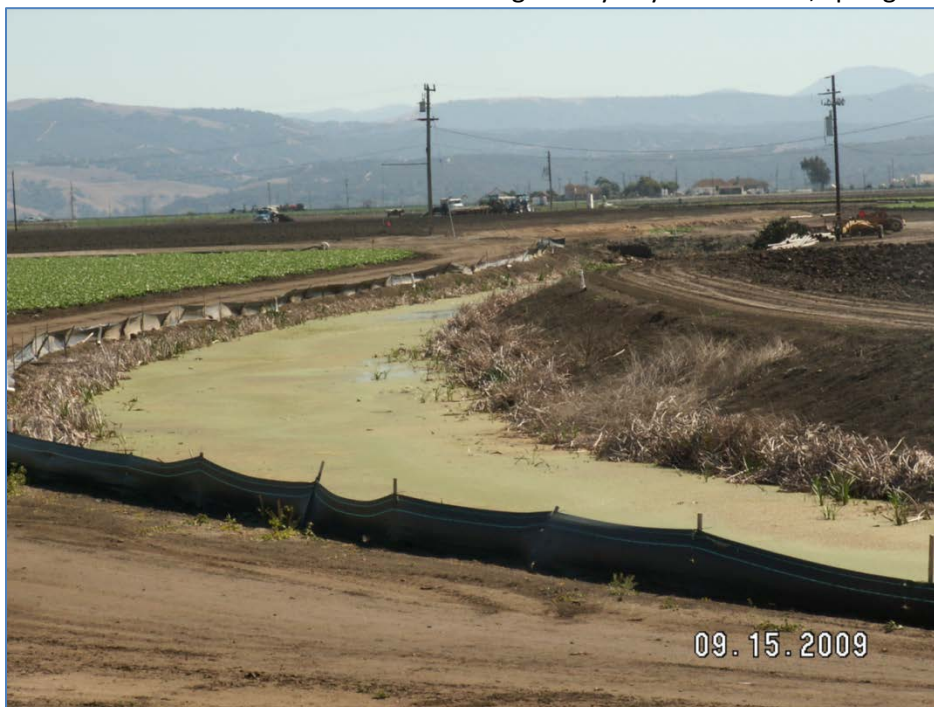
Tembladero Slough before it empties into Elkhorn Slough and the Monterey Bay National Marine Sanctuary, Monterey Co.
