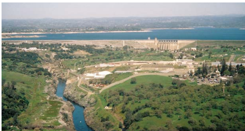
Folsom Dam looking eastward.
