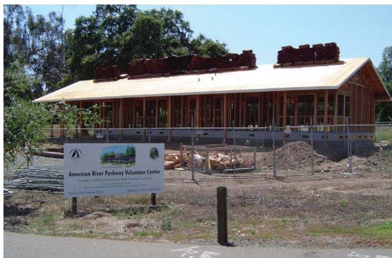
The American River Parkway Volunteer Center in progress.
