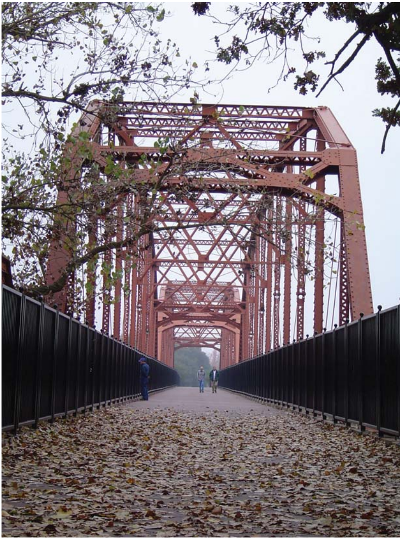
Old Fair Oaks bridge.
