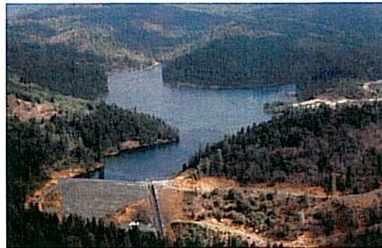
Figure 7 – Sugar Pine Dam and Reservoir
