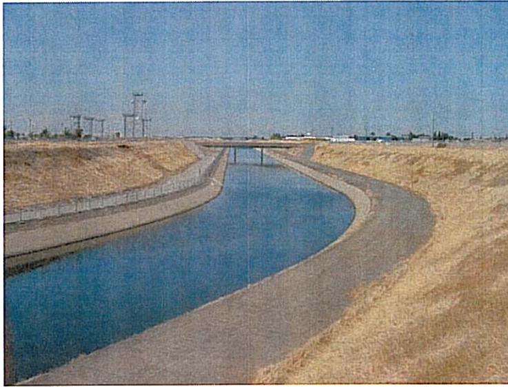
Figure 8 – Folsom South Canal at Douglas Blvd. looking north.
